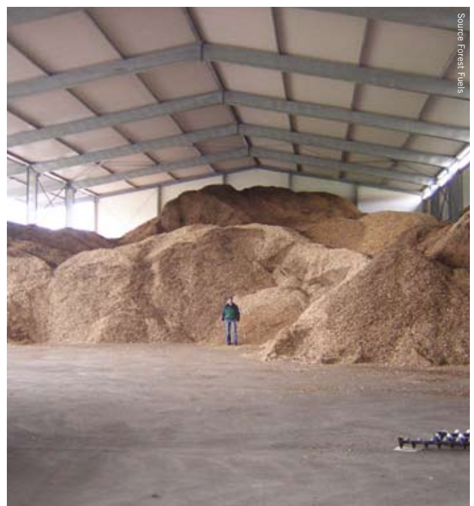
Large scale dry chip fuel store at distribution depot
