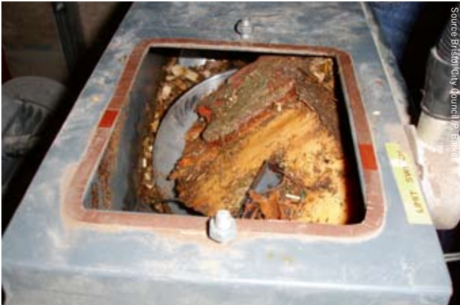
Oversize material causing blockage in feed auger
