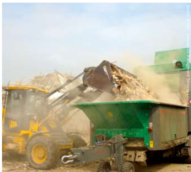
Jenz Shredder being loaded with recycled wood waste at waste transfer station
